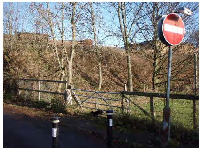
Photograph 4 – Hazel Grove Railway Embankment at Mill Lane looking northeast.
