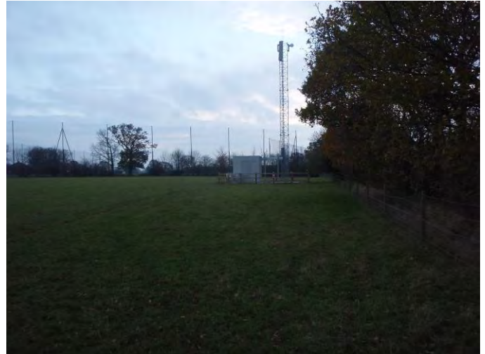
Photograph 32 – Mobile phone mast south of the alignment, east of Styal Railway Line.
