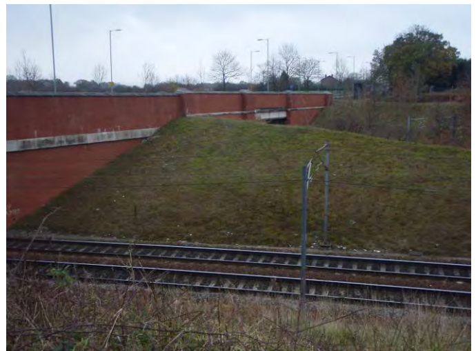
Photograph 37 – Western side of southern Styal Road rail bridge – looking south east
