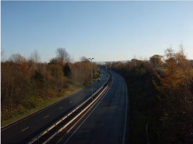
Photograph 25 – Woodford Road junction viewed from footbridge – looking east.
