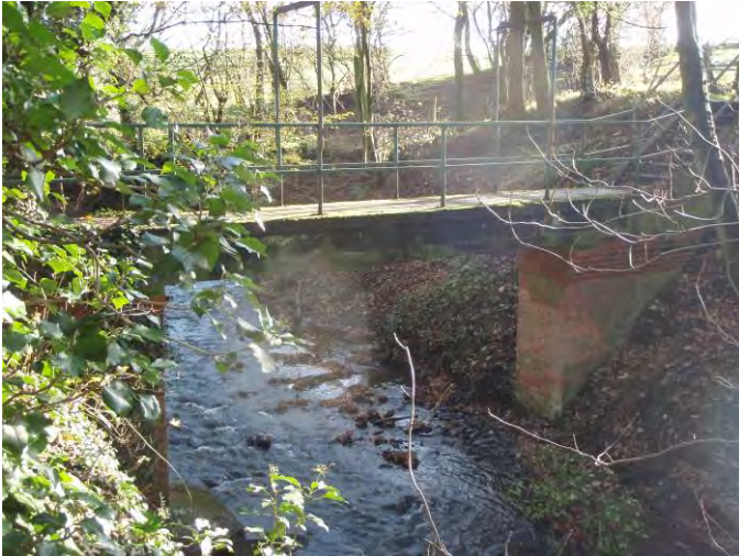
Photograph 9 – Norbury Brook footbridge at Old Mill Lane
