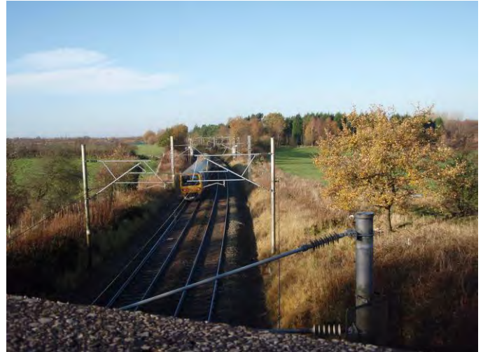
Photograph 15 – view of West Coast Mainline looking northeast from Woodford Road
