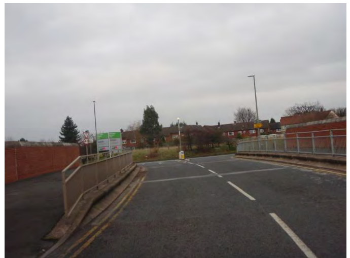
Photograph 41 – Ringway Road Bridge – Looking north.
