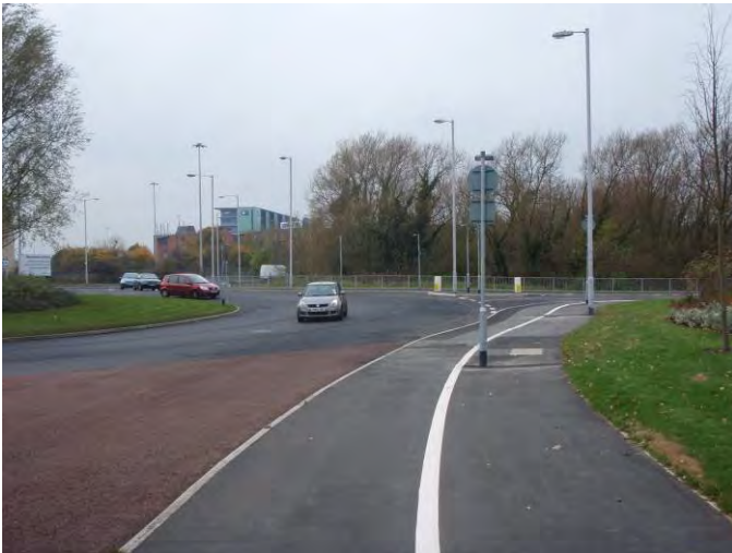
Photograph 43 – Ringway Road West/Aviator Way roundabout – Looking west.
