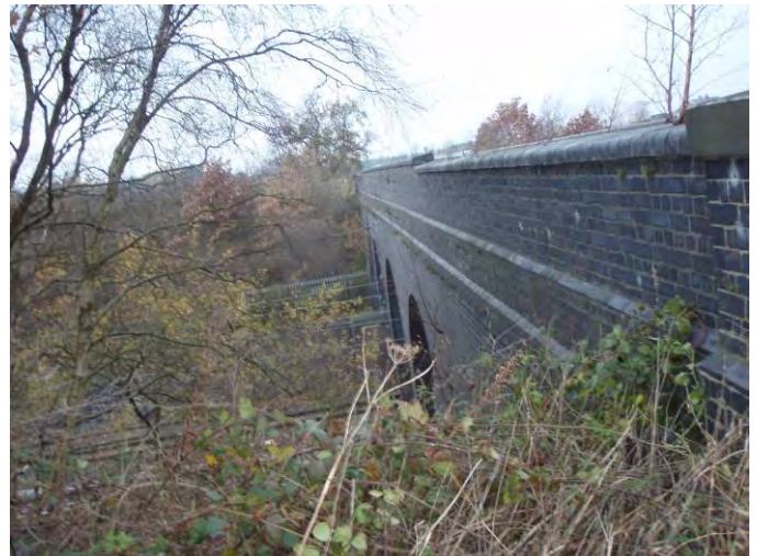
Photograph 33 – Rail bridge and cutting – looking west.
