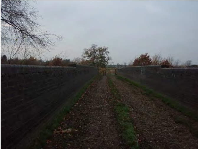
Photograph 34 – Rail bridge – looking west
