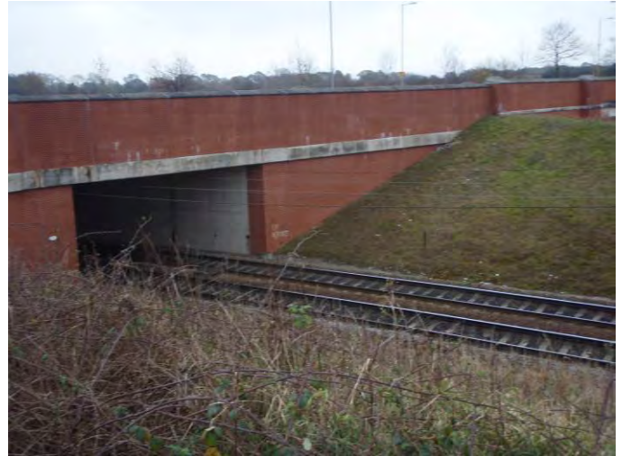
Photograph 36 – Western side of northern Styal Road rail bridge – looking south east
