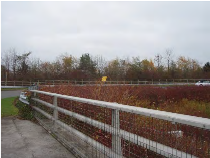
Photograph 47 – M56 Junction roundabout – Looking north from the western roundabout bridge.
