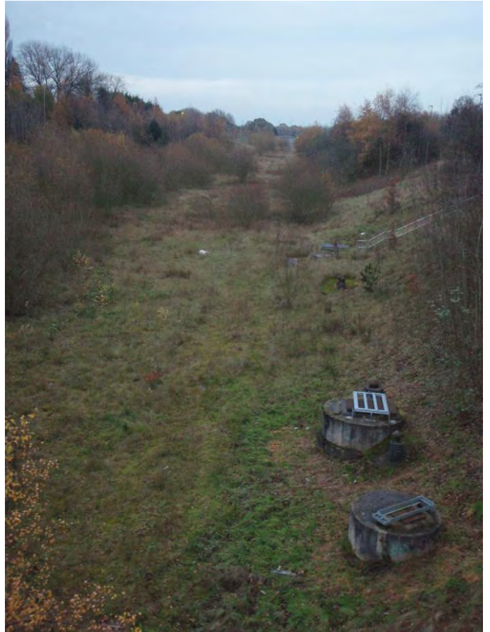
Photograph 29 – A555 looking east from Wilmslow Road bridge.
